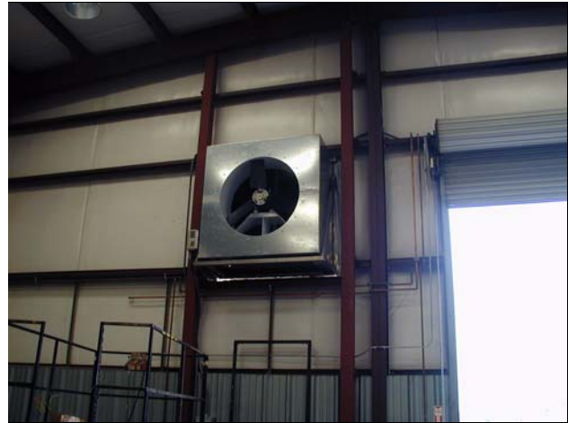
SNAP digital output modules enable a Linux-based controller to regulate the cooler's fans
