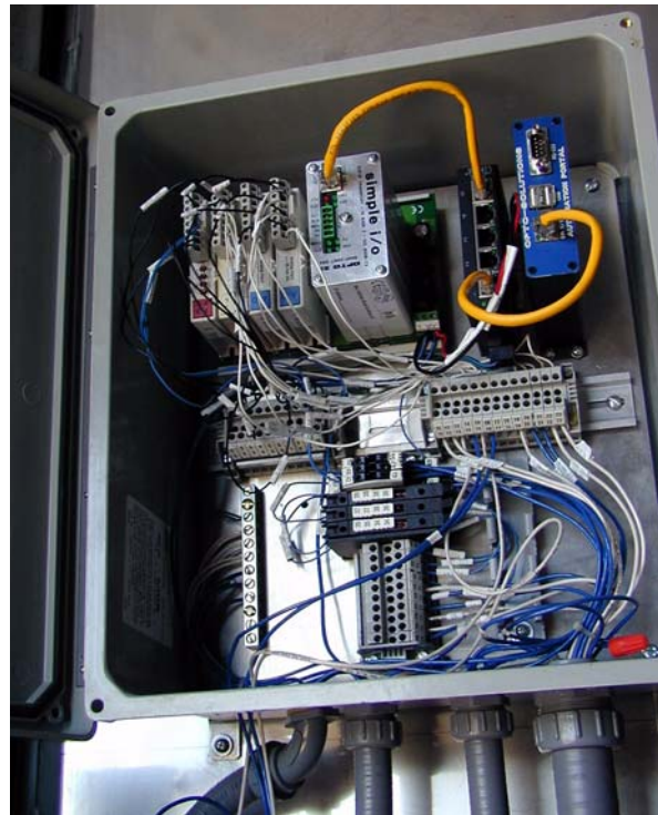
AZFlow coolers have embedded Opto 22 SNAP-brand control hardware as their central component
